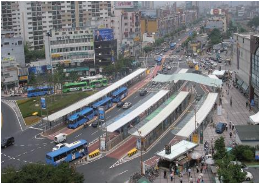
Figure 6. BRT transfer centre at Cheongryangni Station, Seoul
