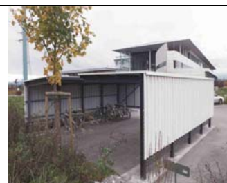
Plate 5: The second cycle stand in the Vorarlberger Medienhaus sends out the right signal, increases capacity and also gives better protection against bad weather.
