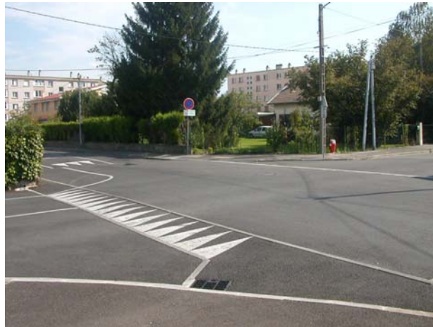
Figure 4.8. Raised junction in Grenoble (France)
