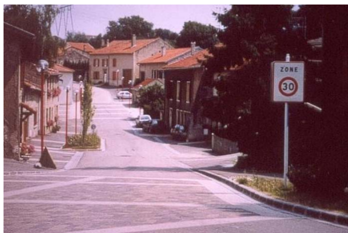
Figure 4.1. Typical design of a 30 km/h zone
