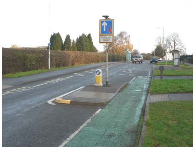
Figure 4.5. Narrowing of a road in Loughborough (United Kingdom)
