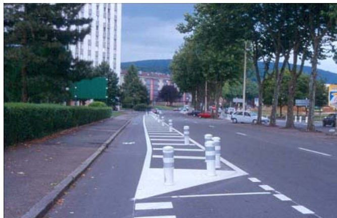
Figure 4.10. Temporary design in Belfort (France)
