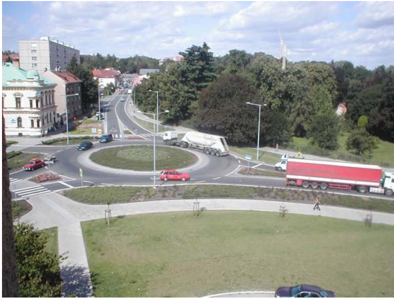
Figure 4.6. Roundabout in Chrudim (Czech Republic)
