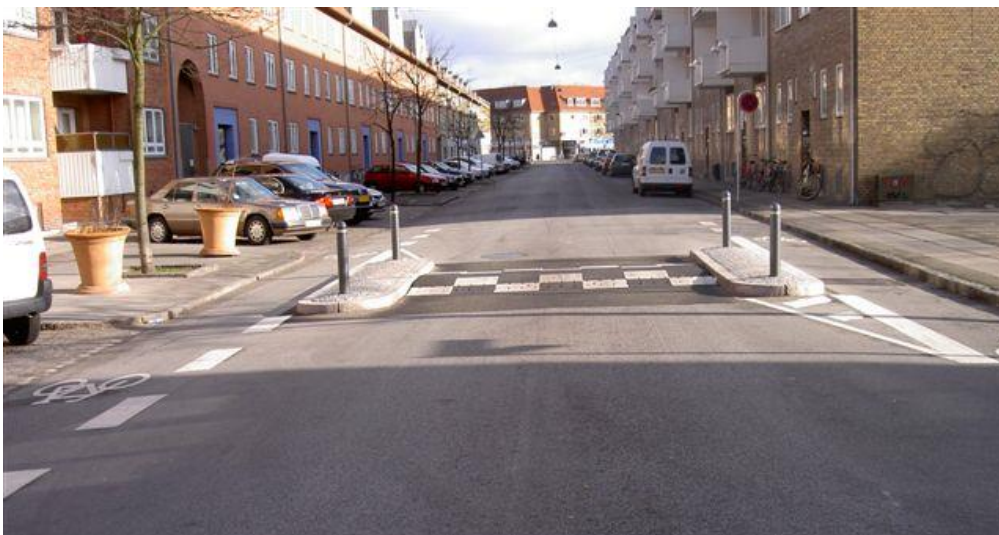
Figure 5.21 Road hump with kerbed islands and bollards
