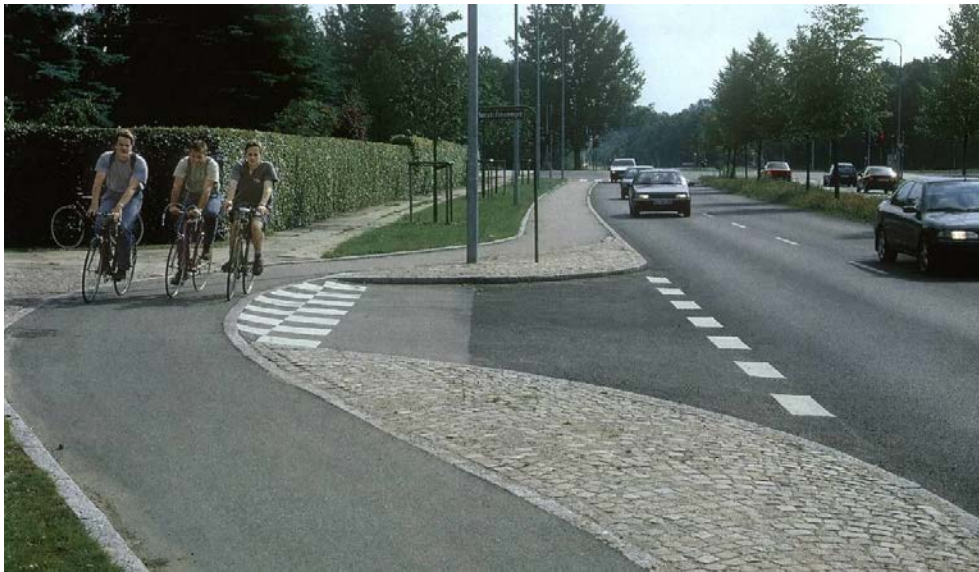
Figure 5.26 Recessed bicycle track
