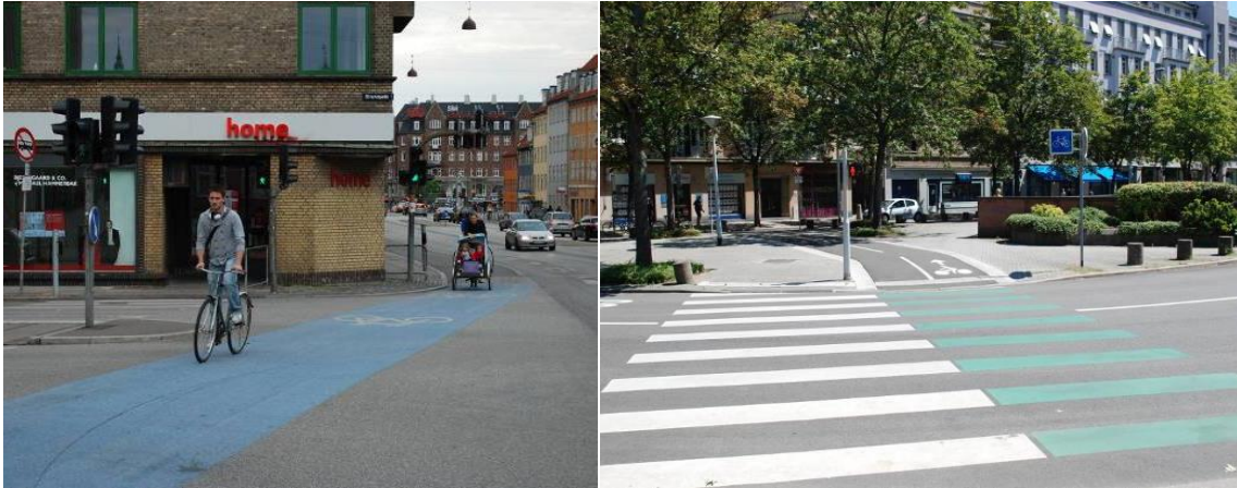
Figure 5.38 Coloured bicycle crossings at junctions
