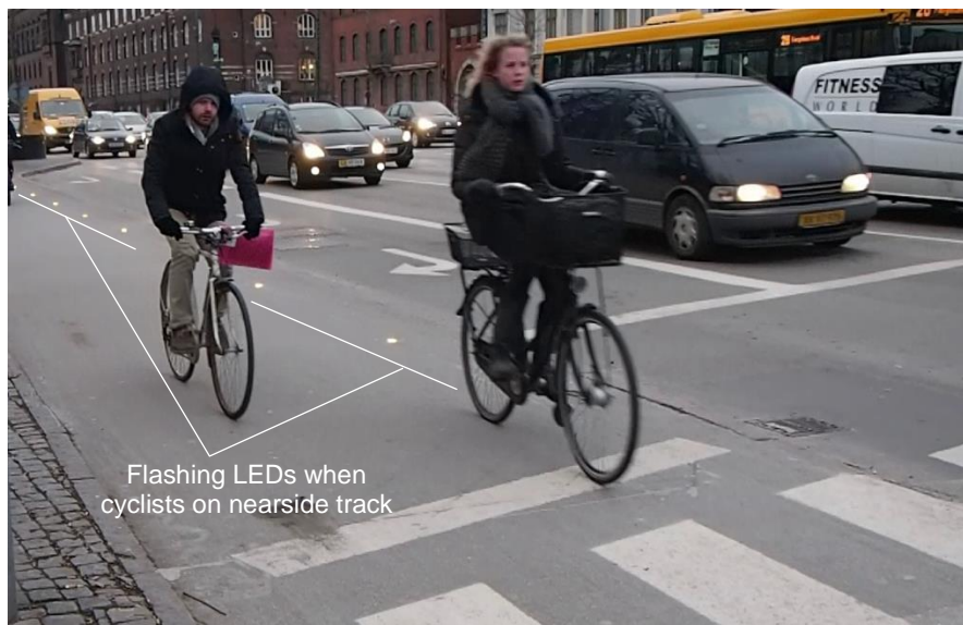
Figure 5.43 Sensor-activated LED lights warning nearside turning motorists of presence of cyclist in nearside bicycle lane (Copenhagen)
