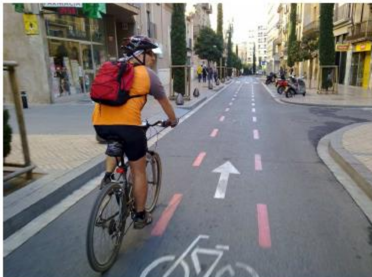
Figure 5.40 Cycle path in the middle of the road
