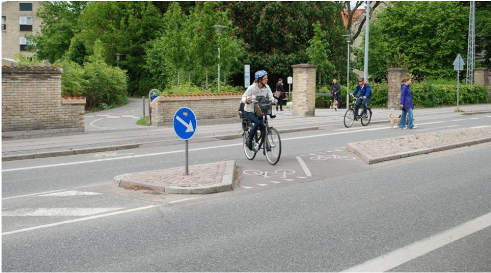
Figure 5.23 Central island at bicycle crossing on urban road
