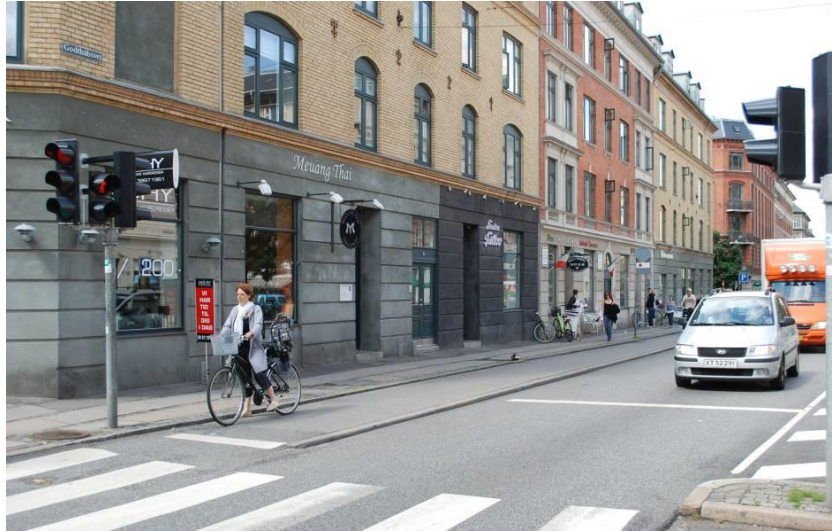
Figure 5.32 Advanced stop line in signalised junction (Copenhagen)
