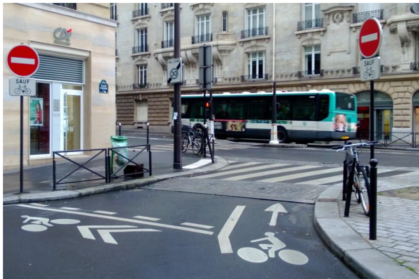
Figure 5.28 Side road entry treatment (SRET) with contra-flow bicycle lane (Paris)
