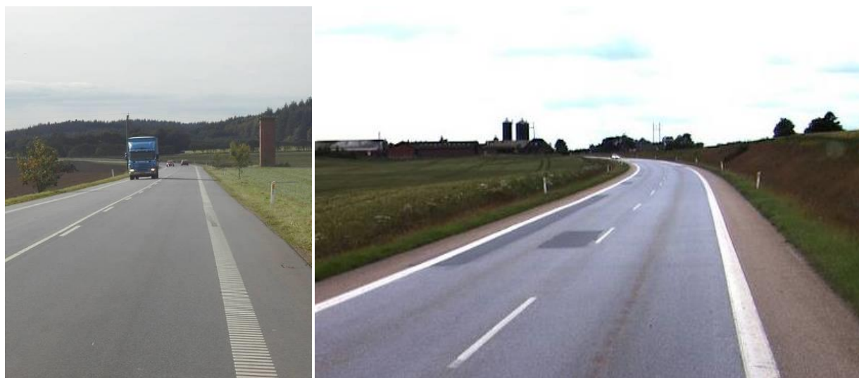
Figure 5.20 Paved shoulders on rural roads (Denmark)
