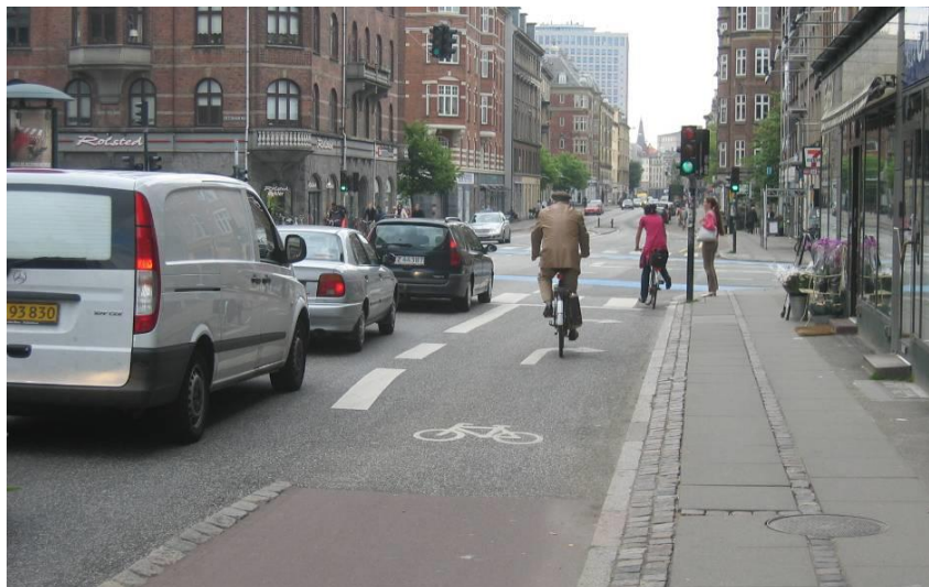
Figure 5.35 Truncated bicycle track in signalised junction (Copenhagen)
