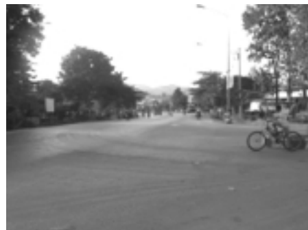
Highway 120 km. 45+400-45+800 (Phayao - Wang Nua): Highway junction without signalizations and insufficient roadway markings.
