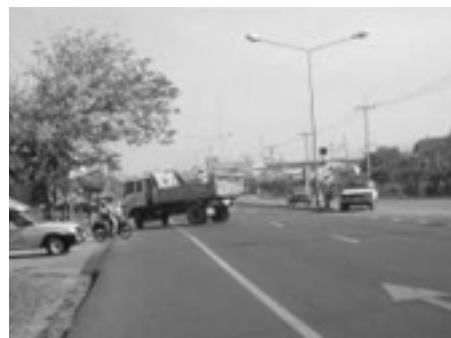
Highway 1001 km. 2+950 ? 2+961 (Chiangmai - Mae Joe): Opening U-Turn with a road junction, where local traffic conflicts with fast through traffic.
