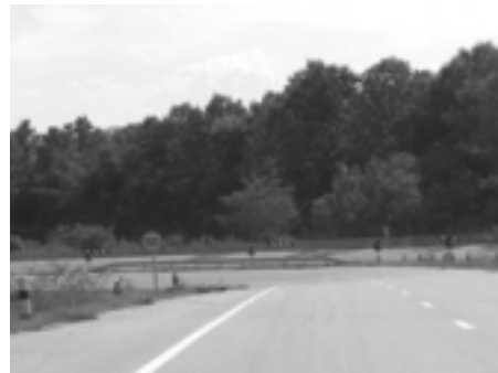
Highway 1 km. 638+435 - 638+500 (Lampang - Chiangrai): 1) Sharp horizontal curve mixed with vertical slope, 2) Speedy traffic with insufficient super elevation.
