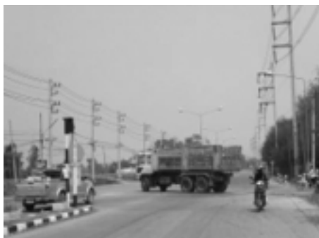
Highway 1035 km. 4+450 - 4+500 (Lampang - Jaehom): Opening U-Turn with a road junction on narrow right of way and poor roadway markings.
