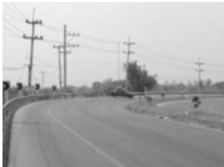
Highway 108 km. 34+100 - 34+200 (Sanpatong - Jomthong): Sharp curve with an opening entrance on slippery surface and no roadway lightings.
