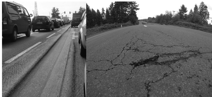
Figure 2.5. Heat damage to asphalt pavements: Rutting and cracking
