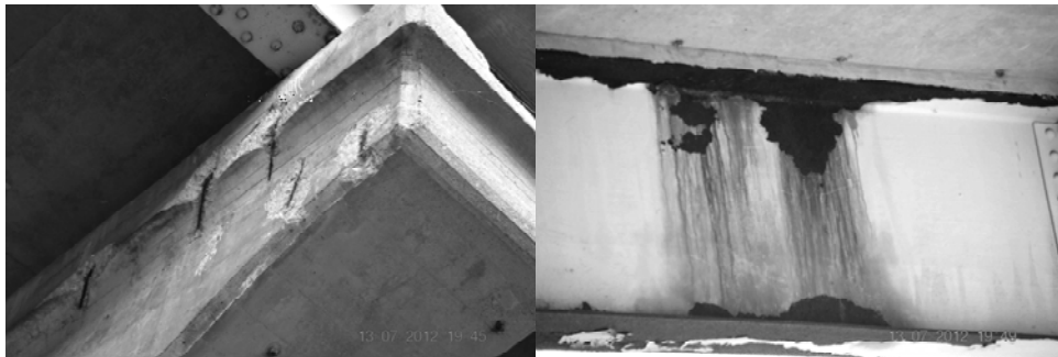
Figure 2.11. Steel and concrete bridge component corrosion
