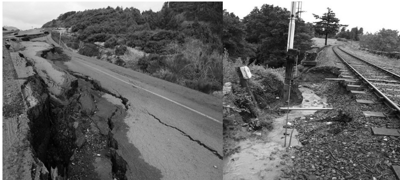
Figure 2.9. Foundation washout and collapse
