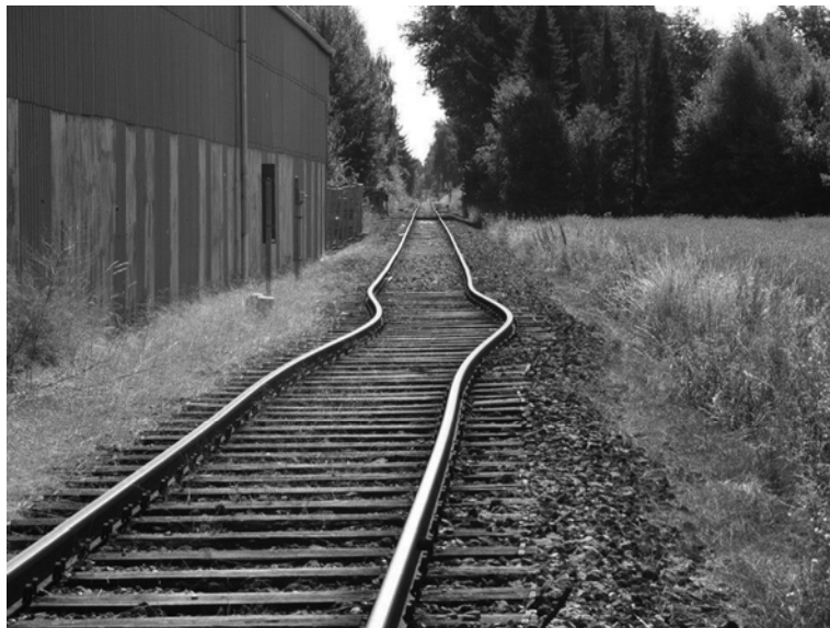
Figure 2.18. Heat-induced track buckling
