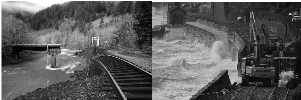
Figure 2.16. Impacts of storm-related embankment scour
