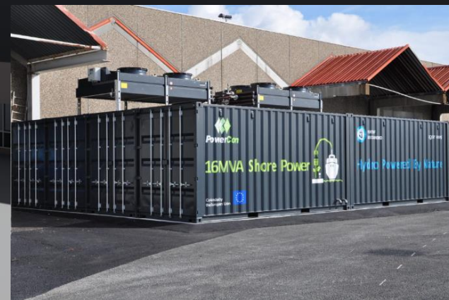
Kristiansand, 16 MVA, one ship at a time
