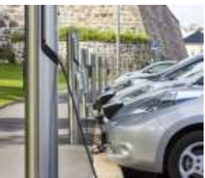
PRIVATE & PUBLIC EVSE ROLLOUT
