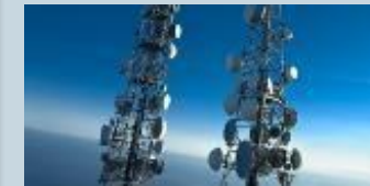
Extended and modernized telecoms infrastructure
