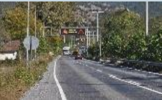
Single Lane Road and Improvement
